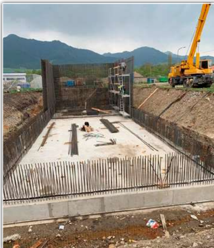
Construction shell of the new wastewater treatment plant in Liptovský Mikuláš.
